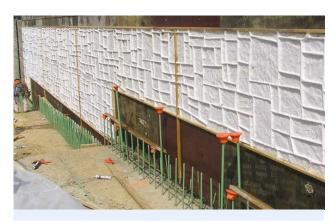
Sika thermoformed plastic formliners are used for texturing tilt- up, cast-in-place or precast architectural concrete. Sheets of formliner attach to the formwork or casting bed prior to placing the concrete. Following placement and normal curing time, the formwork and formliner are stripped, leaving a textured concrete surface.
