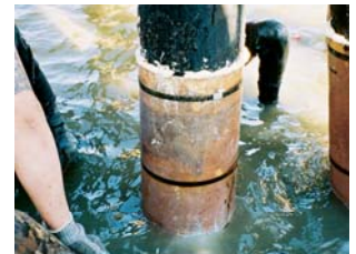
Repaired Pile with Epoxy Mortar
