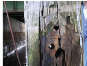
Decayed Timber Pile
