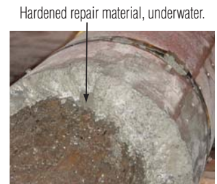
Hardened repair material, underwater. Cross Section of Repaired Pile. Repair Material Thickness = 1.5" - 2"
