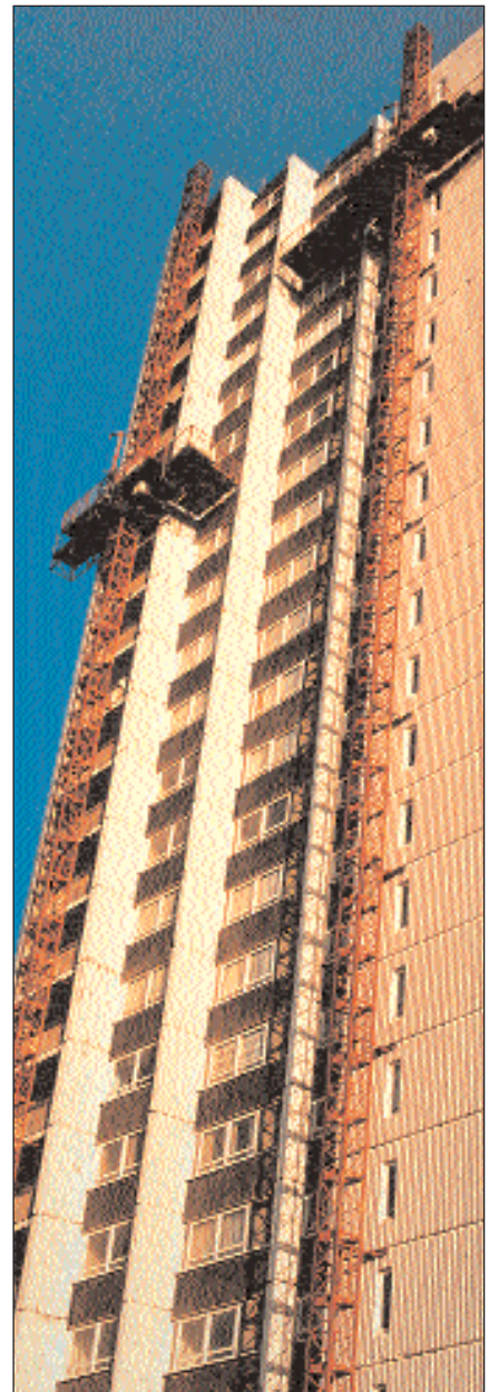
Concrete Repair and Protection Project in Progress
