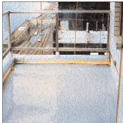
Sikafloor Traffic System on a Private Balcony
