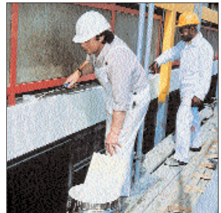
Roller Application of Sikagard Elastocolor
