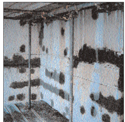
Spalls filled with Sika MonoTop Ready for Leveling and Protection
