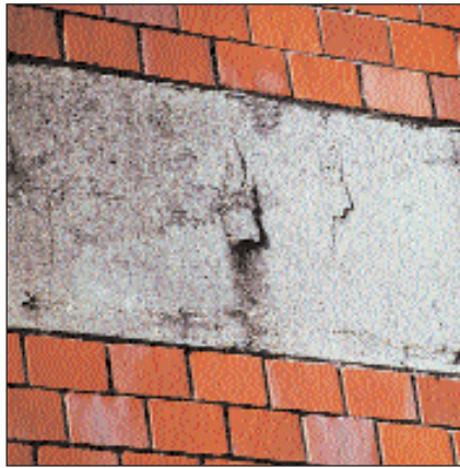
Cracking
