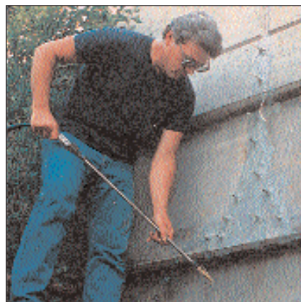
Sikadur Injection System on a Building Facade
