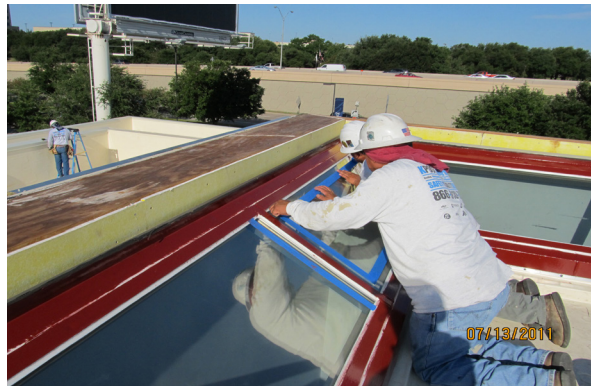
Applied Clearglaze with foam roller
