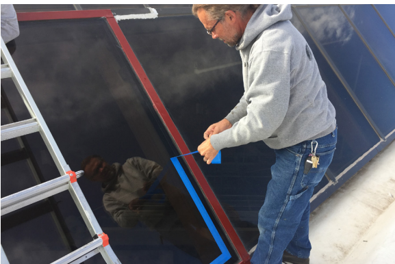
Pull masking tape while 2 nd coat is wet
