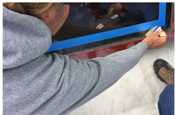
2 nd Application of masking tape to dry primer
