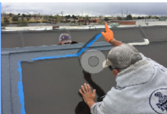
Pull masking tape while 2 nd coat is wet
